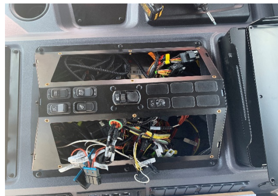
Figure 8: Doghouse w/Panels Removed
