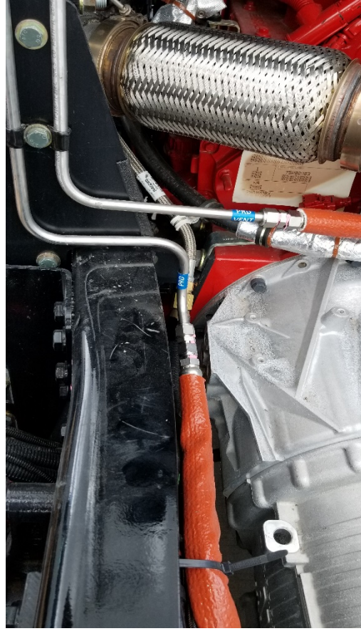
Figure 42: PRD Vent Installation Cont.
