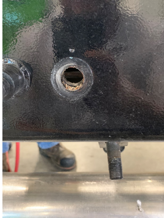
Figure 5: After Huck Removal
