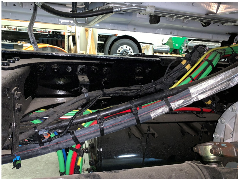
Figure 16: Wiring Harness Routing-Under Cab
