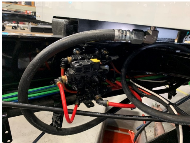
Figure 37: Low Pressure Fuel Line Install
