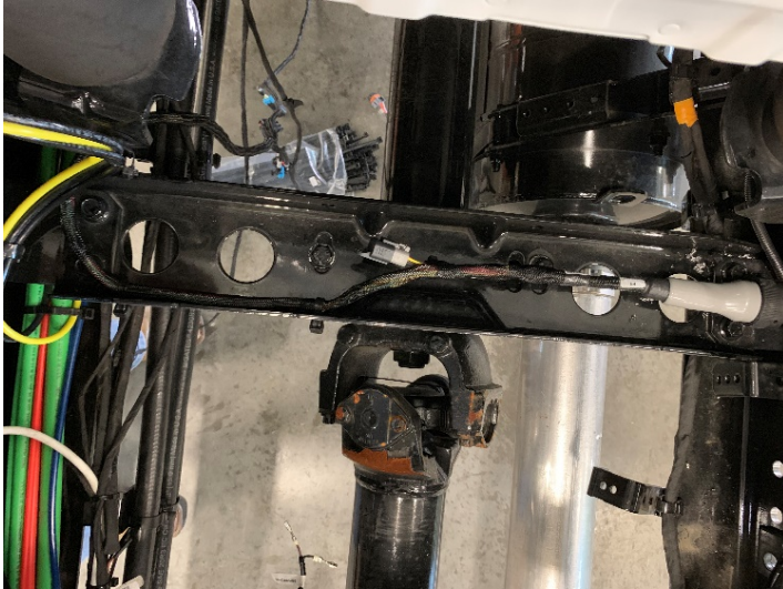
Figure 23: BOC Harness Install
