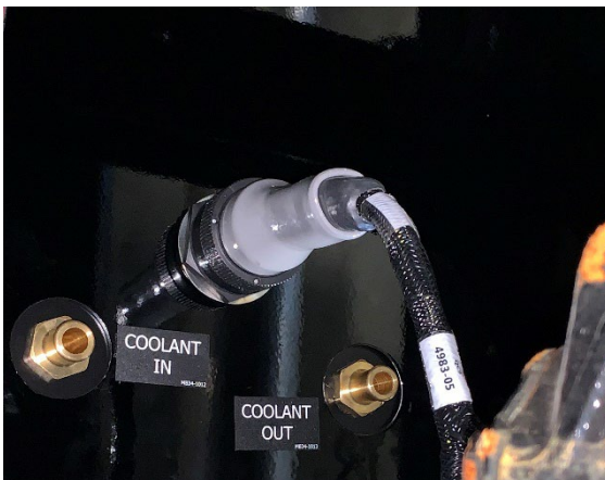
Figure 17: BOC Electrical Connection
