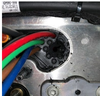
Figure 6: Firewall Hole Drilled
